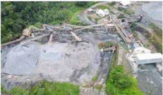
Finally, these final products would be transported to a cement plant 3.5km away via this overland conveyor.
